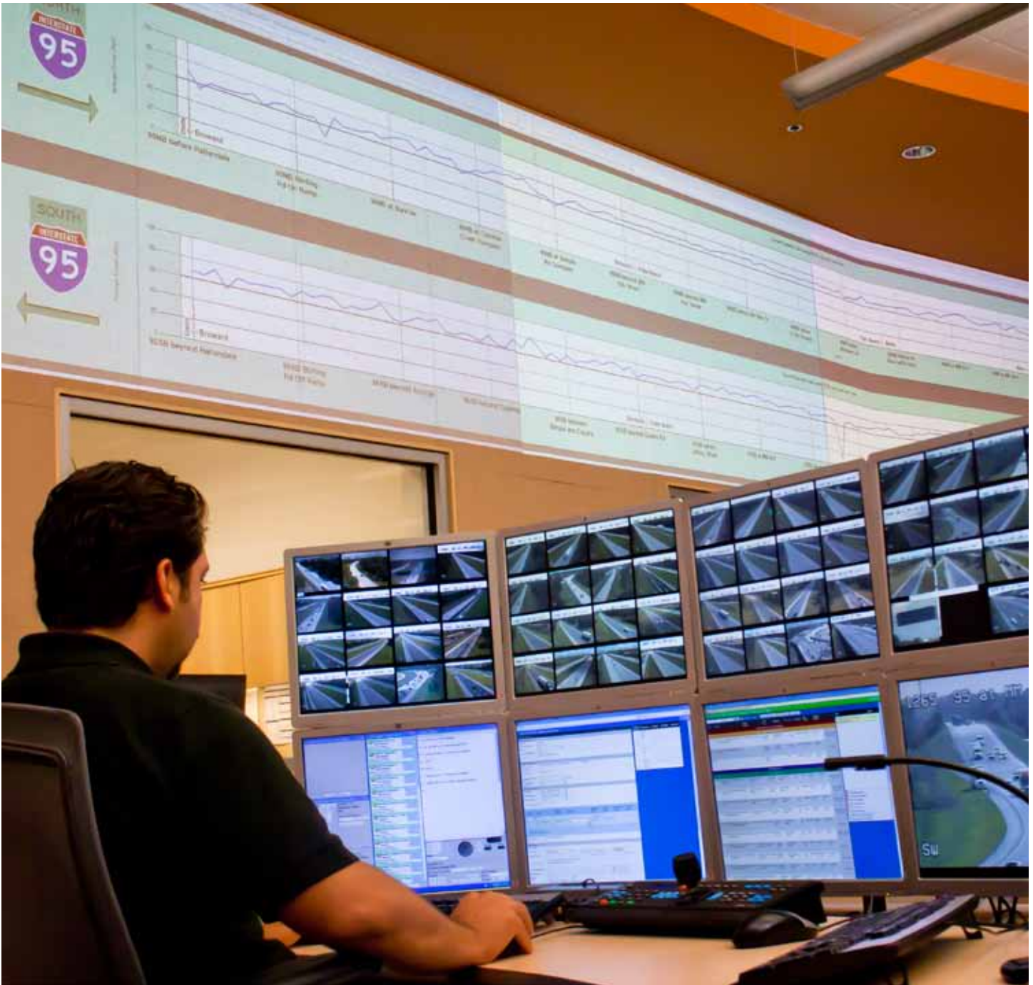
Real time speed data charts are displayed on unused wall space in the control room to give operators another tool to monitor traffic.
